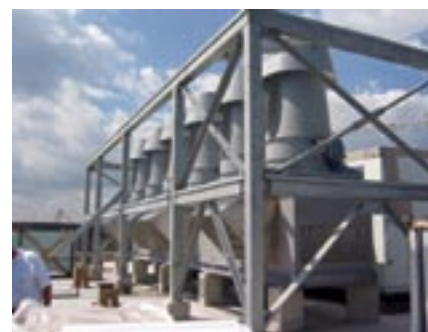
Photo 1: Mixed-flow impeller systems on the roof of the Toronto Medical Discovery Tower
