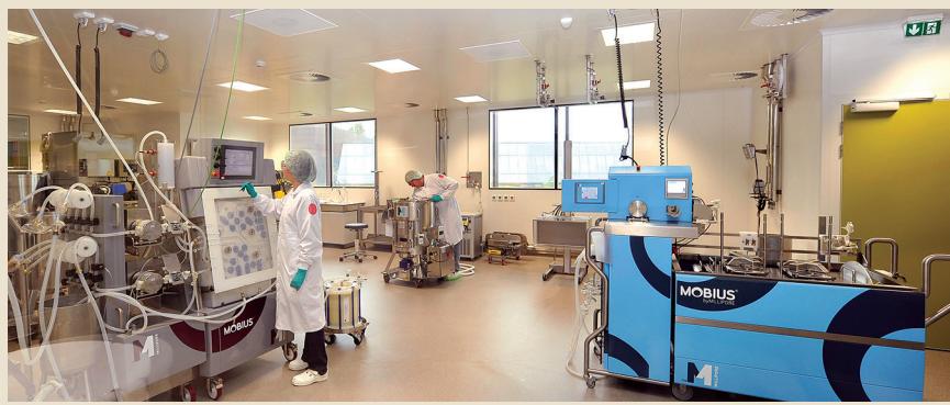
Photo 2: Downstream processing area with the Mobius FlexReady chromatography system (left) and customized Mobius FlexReady system for viral filtration (right); equipment is connected from the ceiling (power supply and network).
