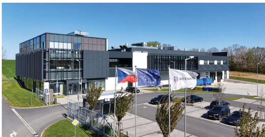
Brenntag Pharma good manufacturing practice (GMP) hub with dedicated class C cleanrooms for biobuffer manufacturing. ( HTTPS://WWW.BRENNTAG.COM/EN-GB/INDUSTRIES/PHARMA/PHARMA-GMP-HUB )
