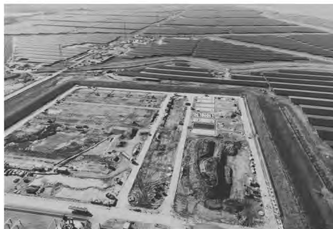
The Cleve Hill solar and BESS project under construction. Image: Quinbrook Infrastructure Partners.
