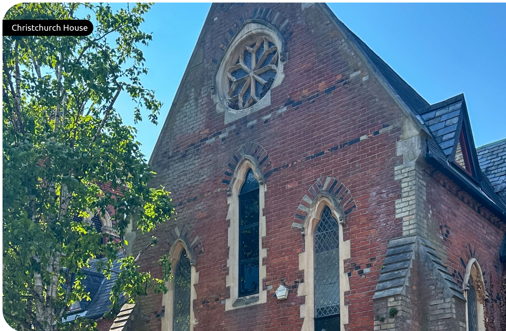
Former Cardigan Street Chapel
