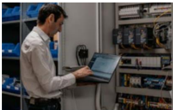
Image ME_BHB_02: Thanks to a digital twin, the washing system can be thoroughly tested at the desk. This drastically reduces the commissioning time.
