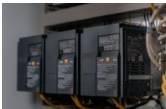
Image ME_BHB_03: Mitsubishi Electric's FR-E800 series frequency inverters enable energy-efficient control of brushes and pumps.
