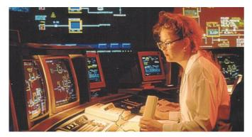
The new system utilises standard hardware and open operating systems to allow the equipment to be upgraded using non-specialist personnel, as the system develops over the years. This project is expected to save Wessex Water about £750,000 a year, and is made possible by using a cost-effective combination of small telemetry outstations, low-cost Mitsubishi Electric PLCs and standard PCs running Widows NT.
