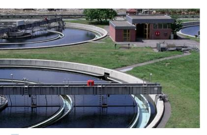
tanks. Here, the microorganisms settle at the bottom of the tanks as sludge, which is pumped back to the activated sludge tanks.
