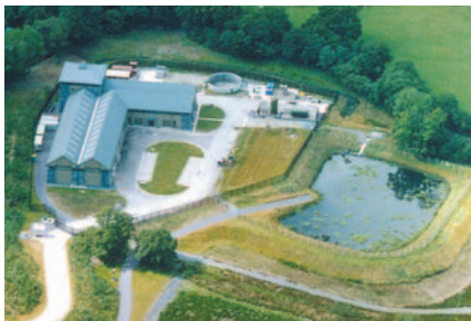
Example of remote pumping station.
