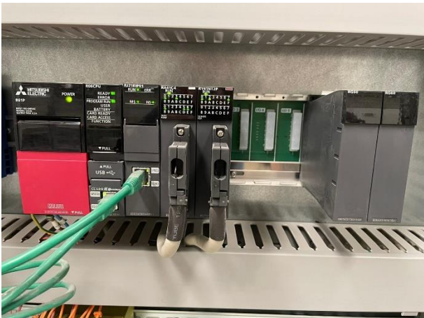
Image 5: To control the 19 VSDs, Profile Developments selected Mitsubishi Electric's iQ-R series PLC.
