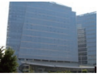
Guangzhou FA Center MITSUBISHI ELECTRIC AUTOMATION (CHINA)LTD.
