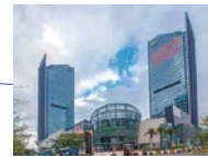
Shenzhen FA Center MITSUBISHI ELECTRIC AUTOMATION (CHINA) LTD.
