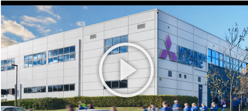
Customer Mitsubishi Electric Air Conditioning Systems Europe Livingston Production Facility - Scotland, UK
