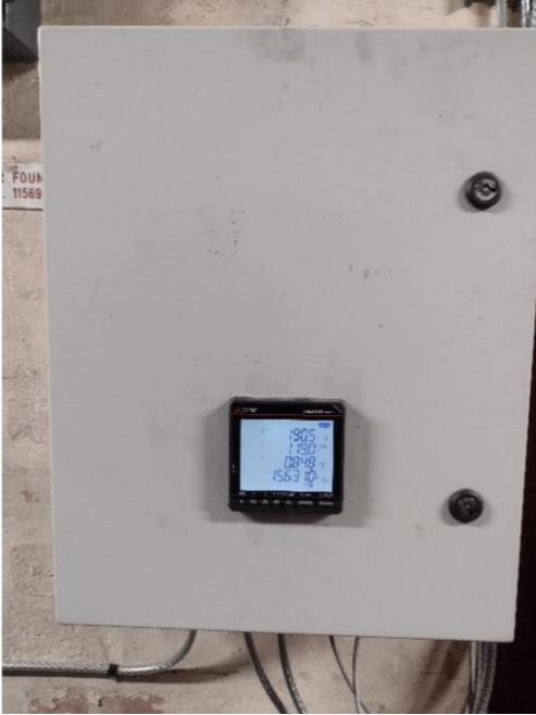
Image 1: Mitsubishi Electric selected the ME96 series of electronic multi-measuring instruments as meters
