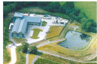
Example of remote pumping station.
