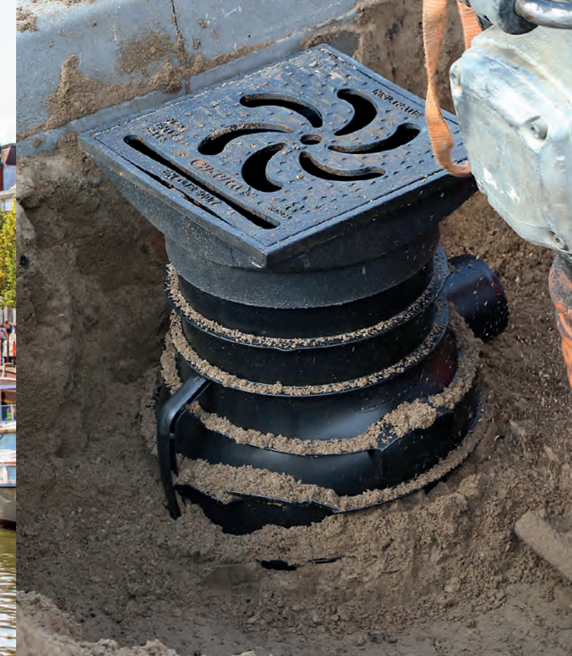
Installation of a Tegra Road Gully.
