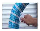
Figure 21: Always protect pipe ends
