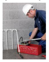
Note: Pressure testing is NOT a substitute for making sure the pipe has been correctly inserted into the Hep<sub>2</sub>O fittings. This should be achieved by following the correct jointing procedure and wherever possible, checking the joints using Hep<sub>2</sub>O joint recognition technology as detailed (see page 18).
