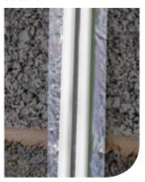
Note: Self adhesive information labels should not be applied directly to Hep<sub>2</sub>O pipes and fittings, they must be placed on suitable surfaces adjacent to the pipe run.
