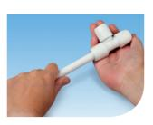
Tug back on the pipe to ensure the grab-ring engages correctly and prevents the pipe withdrawing
