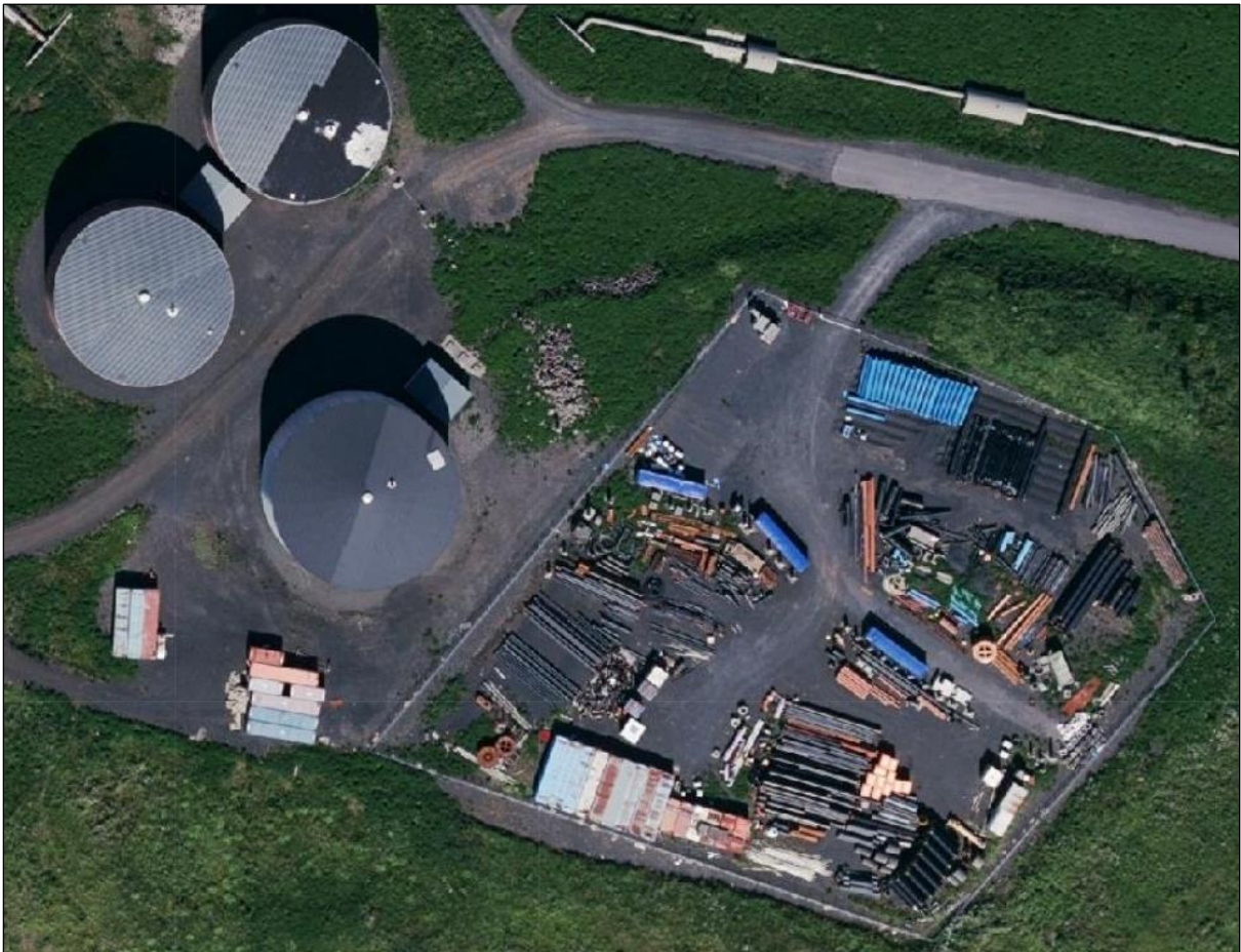
Figure 26. Storage facility at Reynisvatnsheiði.
