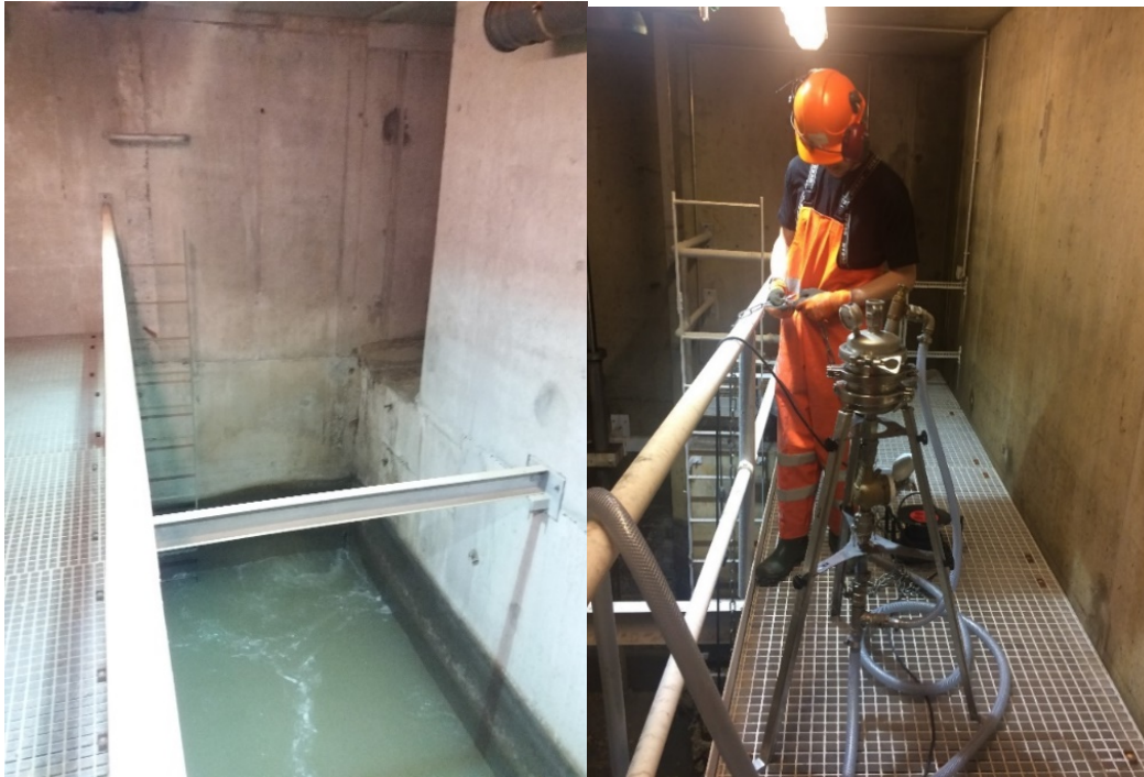
Figure 2 – Example of a sump; filter stack
