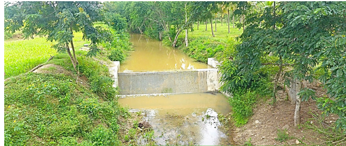
Check Dam in Irudhukottai Cluster, Hosur India
