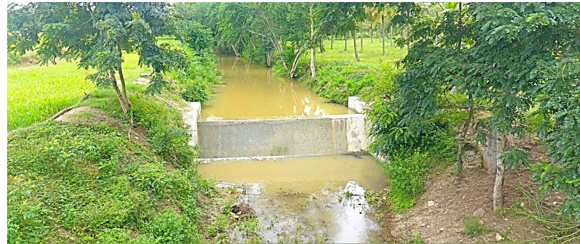
Check Dam in Irudhukottai Cluster, Hosur India
