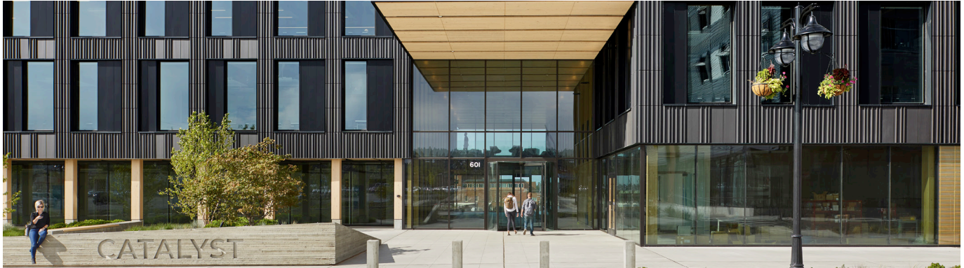
Catalyst | Photo credit: Ben Benschneider | Michael Green Architecture
