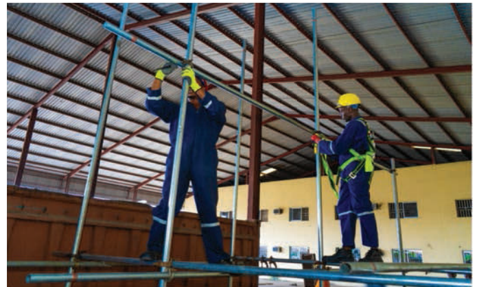
Practical Session with Scaffolding/Rope Access Trainees
