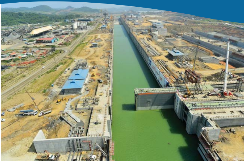
Gate testing, July 3, 2015
