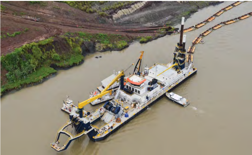
Biggest cutter suction dredger Quibian 1 arrived at the Panama Canal in 2011
