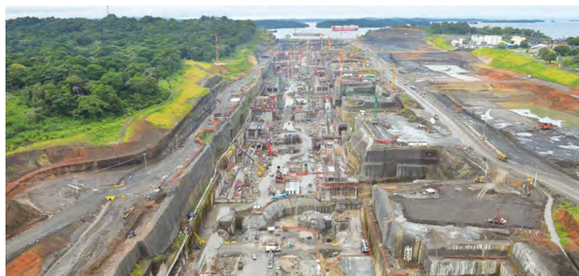
Atlantic site locks construction aerial view from north-to-south
