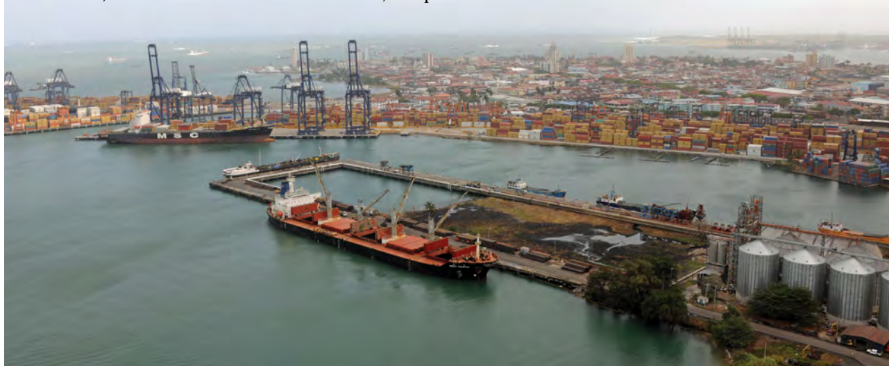
At Cristobal, Talleres Industriales has more than 12,000sq mtr of facilities
