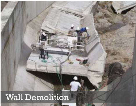
Wire Saw Equipment at GUPC
