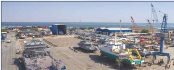
Overview of Repair Bays
