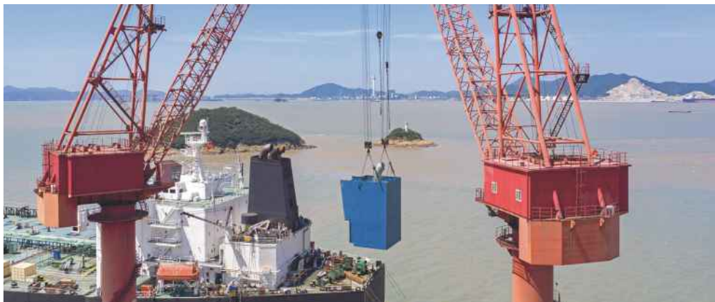
Installing an ENVI-Marine scrubber from Pacific Green Technologies
