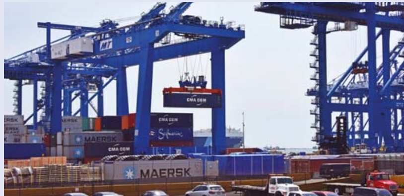
MIT's Automatic Stacking Cranes (ASCs)
