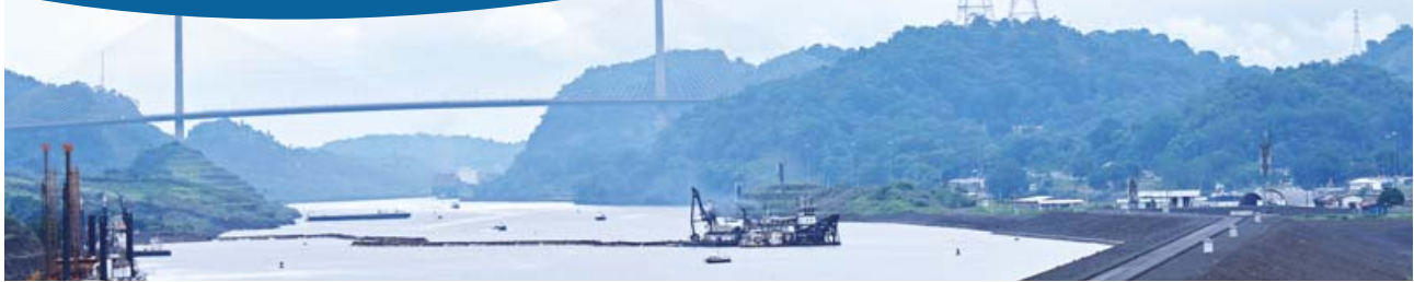
Dredging Pacific access channel at the entrance of new Cocoli Locks
