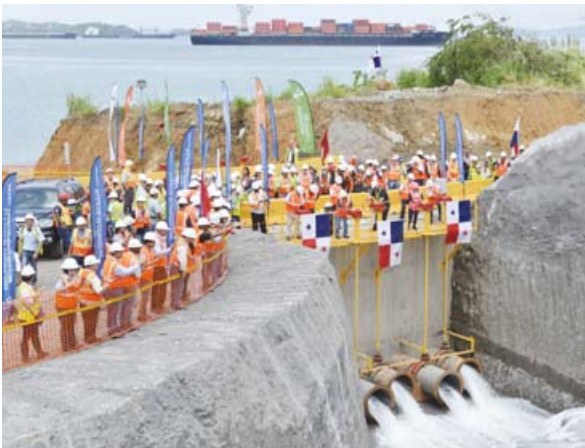
June 11, 2015 – workers witness water flowing into the locks for the first time since works started in 2009
