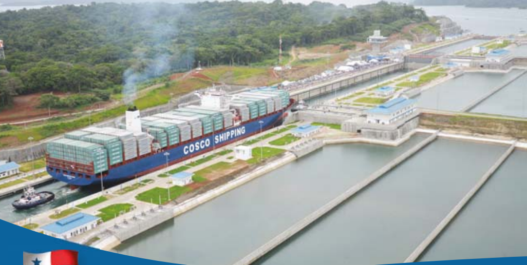
Inauguration of the expanded Canal on June 26, 2016 with the passage of the Cosco Shipping Panama. More than 30,000 people were in attendance
