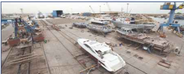
Overview of Repair Bays
