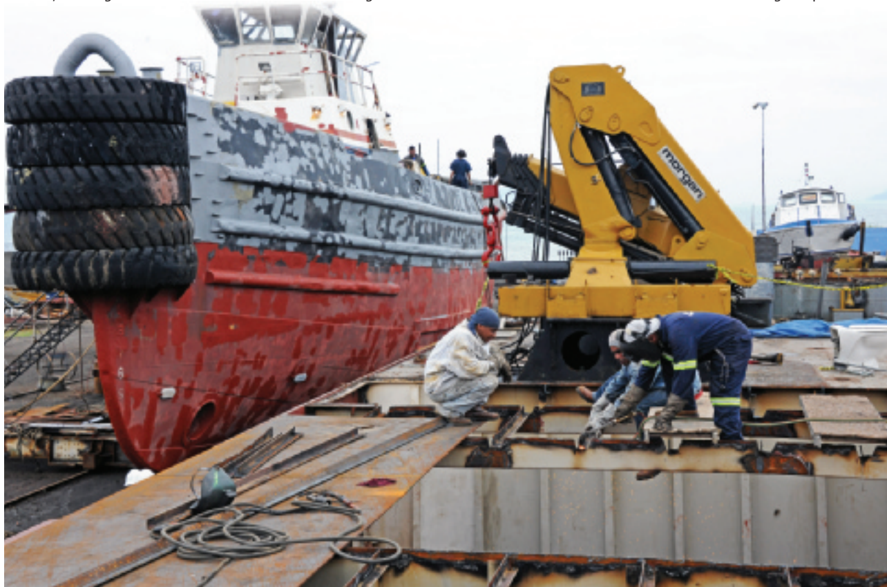
MEC Shipyards – new buildings and repairs
