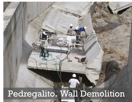
Wire Saw Equipment at GUPC
