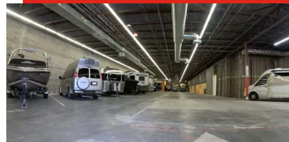
Figure 3 Mixed Use Boat and RV Storage Facility—Conversion from a K-mart
