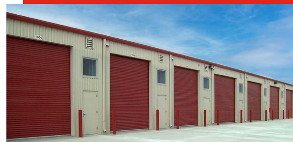
Figure 4 Fully Enclosed Facility
