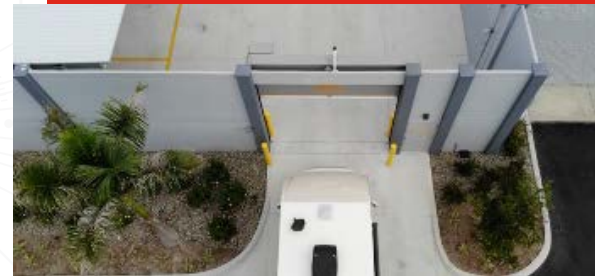
Figure 2 Concrete Barrier Wall Around Canopy Covered, Paved Outdoor Storage
