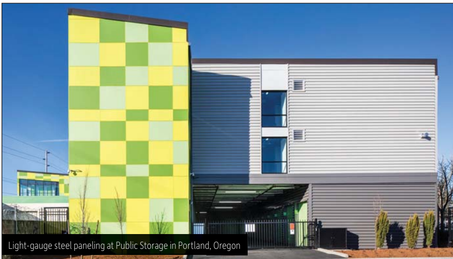
Concrete-masonry units combined with light-gauge steel at Public Storage in Portland, Oregon
